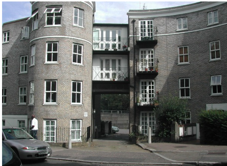
The route into the modern flats' car park marks one end of Riseholme Street, opposite Victoria Park
